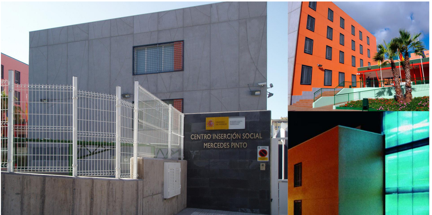
reinforcement concrete structure
